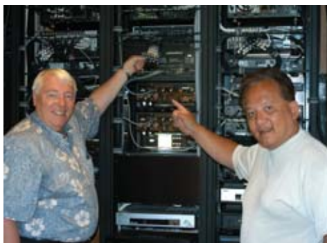
Noel's Home Equipment Rack
